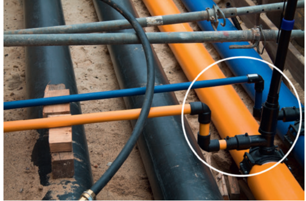
Figure 6.10 Gas pipes and fittings for gas pipes can be made of PA11. This material is the first high-performance polyamide that has been approved to be used for pipes up to 100 mm (4 inches) in diameter at operating pressures up to 14 bars. This material may be biobased and contain 100% renewably sourced ingredients by weight.
